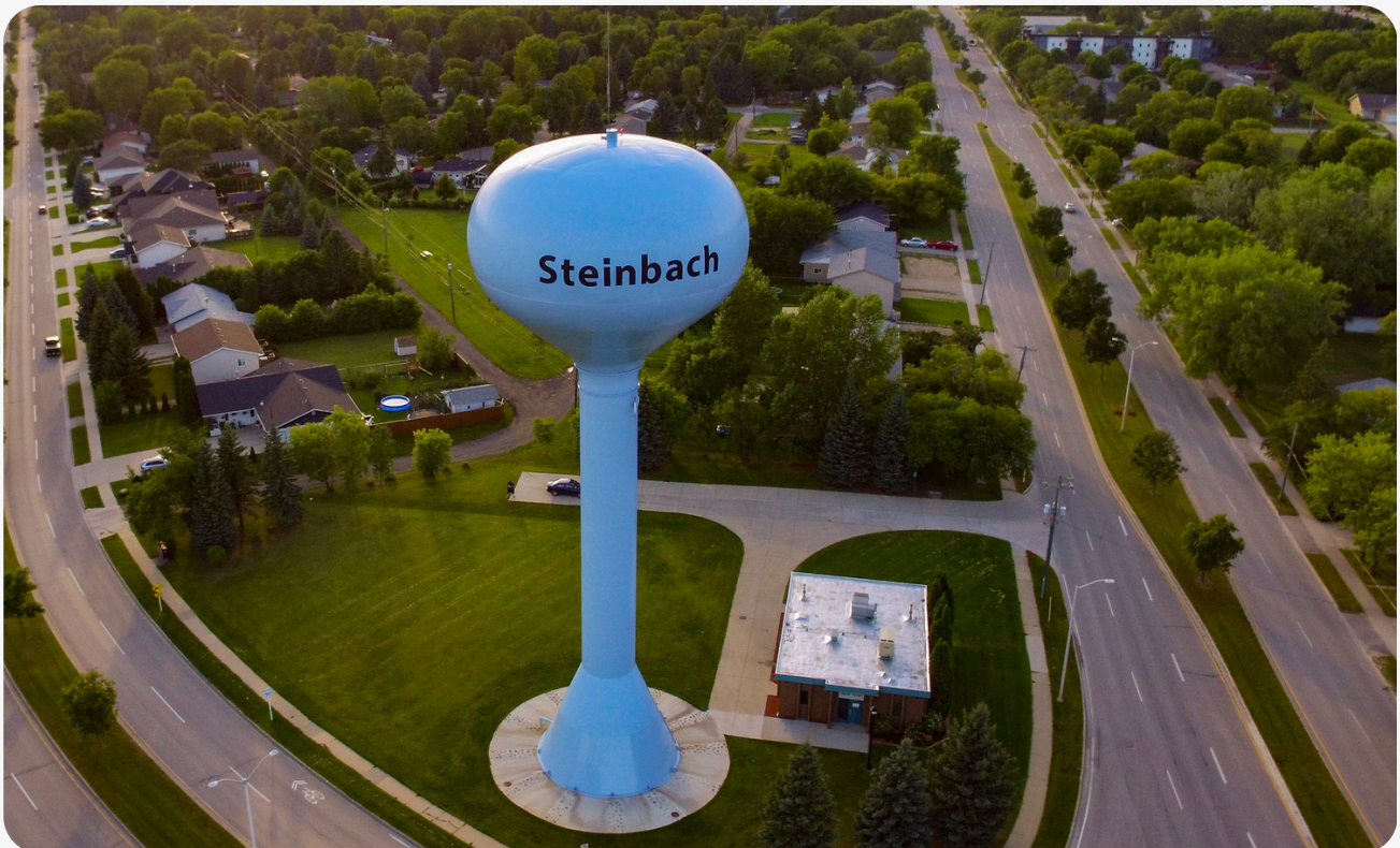
Photo: Aerial shot of Steinbach, provided by City of Steinbach
